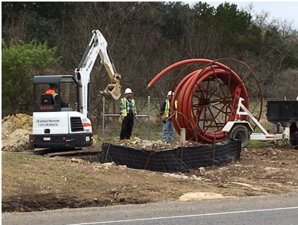
3. TWC Relocation Bore South of Old Black Colony across FM 1626
