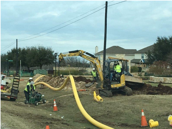
1. Centerpoint Gas Relocation North of Coldwater Hollow
