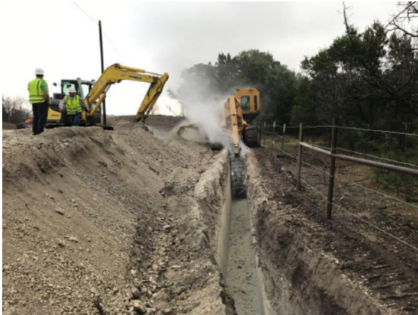
2. Centerpoint Gas Trenching North of FM 2770
