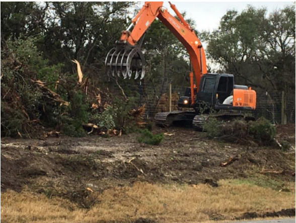
3. C-3 Environmental Brush Removal Westside of FM 1626 at Mustang Creek
