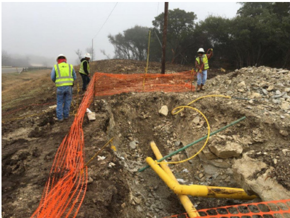
1. CenterPoint Relocations South of Mustang Creek
