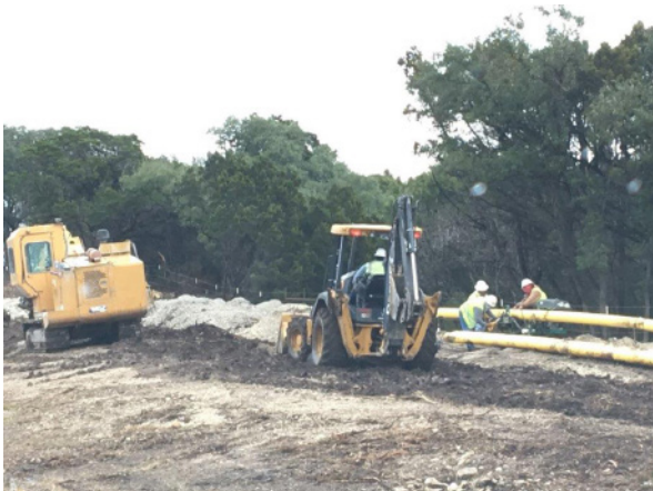
1. CenterPoint Relocations South of Mustang Creek
