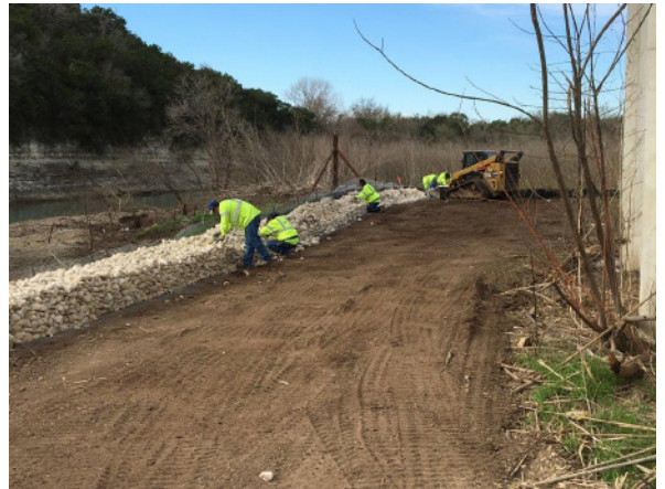
4. BMP Specialist Installing Rock Filter Dams Along Onion Creek
