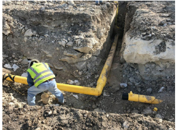
2. Centerpoint Gas Line Tie-in North of FM 2770
