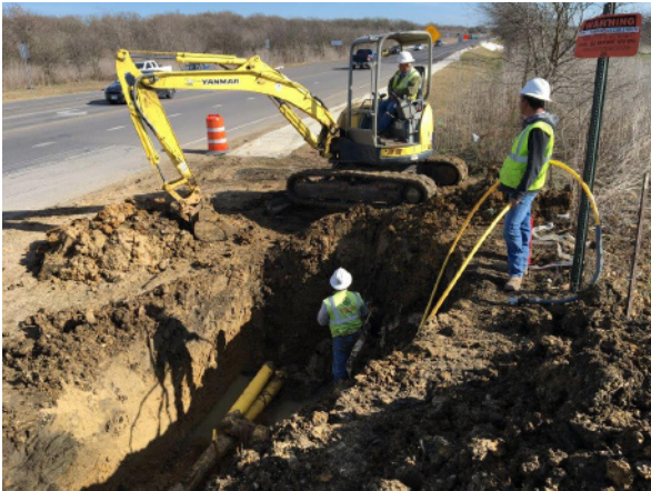
1. Centerpoint Gas Line Tie-in at RM 967
