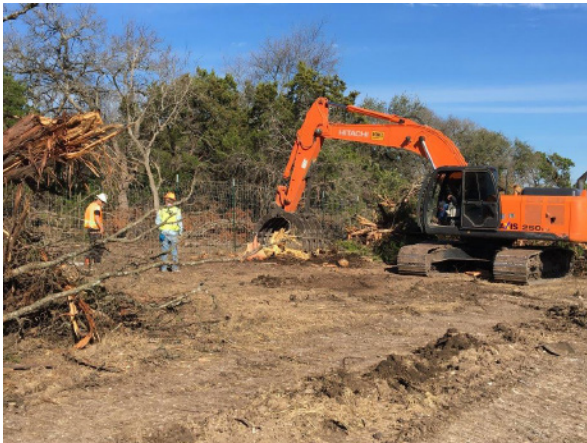
3. C-3 Environmental Brush Removal North of FM 2770 Westside of FM 1626
