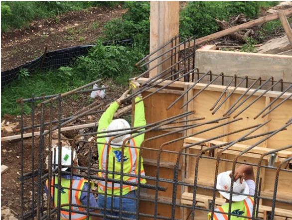
1. Sterling Forming for Proposed Box Culv N of Onion Crk
