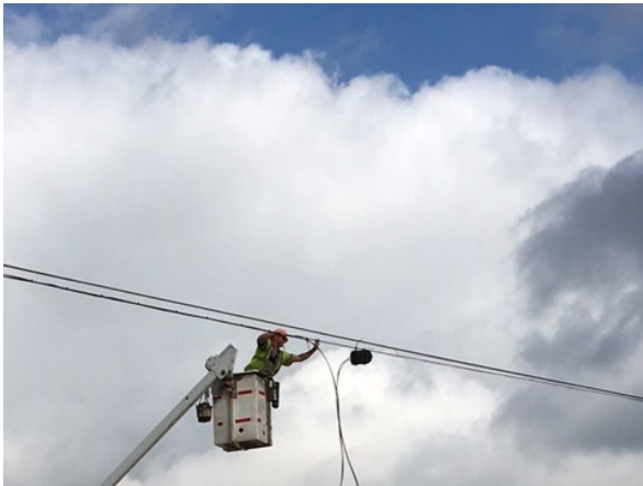
3. Frontier Splicing Fiber North of Mustang Crk
