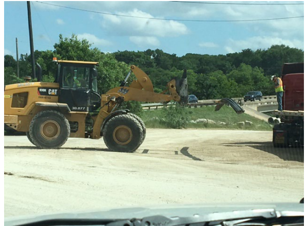
2. Sterling Unloading Steel for Drill Shaft at Mustang Crk
