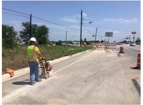
2. TRP Removing Existing Striping N of RM 967
