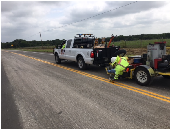
3. TRP Placing Striping N of FM 2770
