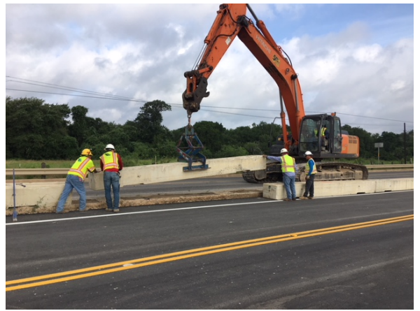
6. Sterling Relocating Concrete Barrier for Traffic Switch N of Onion Creek
