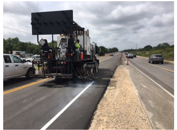
4. TRP Placing Striping N of Cole Springs Rd
