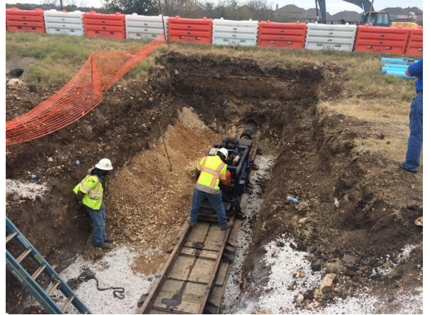
2. City of Buda waterline installation north of Hy Rd
