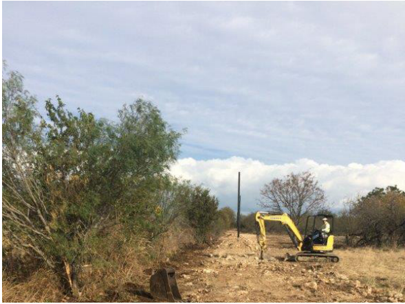
3. Frontier pole installation south of RM 967
