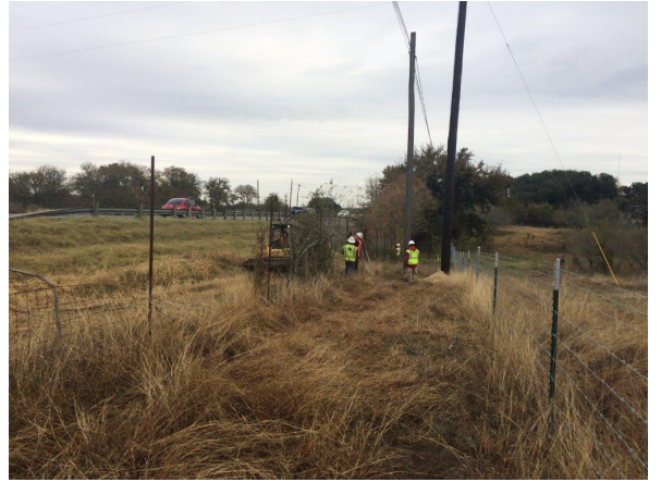
4. Small fence removal north of Onion Creek
