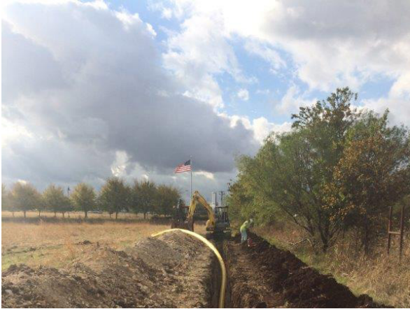
1. Centerpoint Gas relocation north of Oyster Creek
