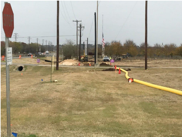
1. Centerpoint Gas relocation south of Oyster Creek
