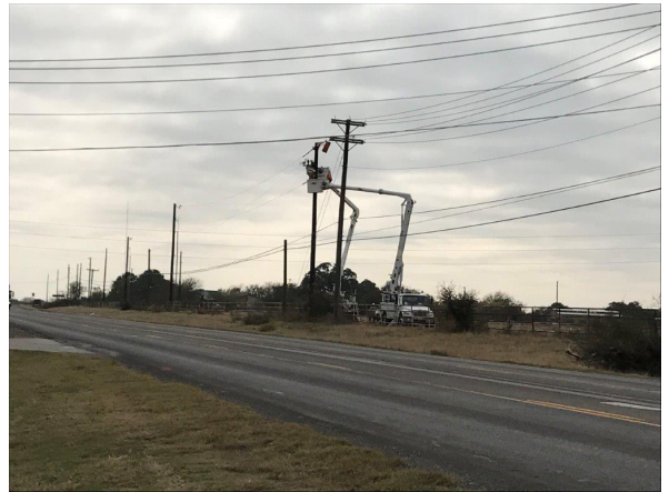
4. PEC relocation across from Elm Grove subdivision
