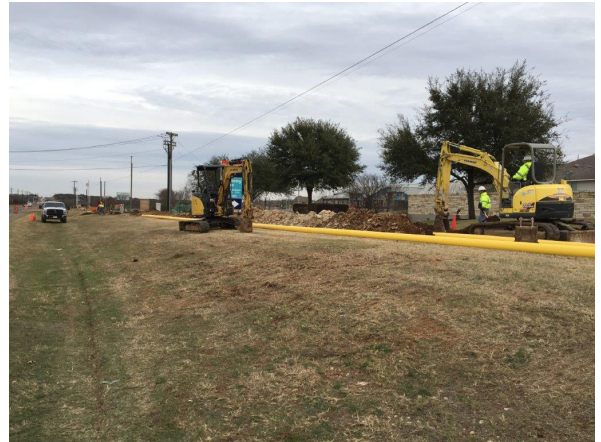
2. CenterPoint Gas Relocations South of Elm Grove Elementary Eastside of ...
