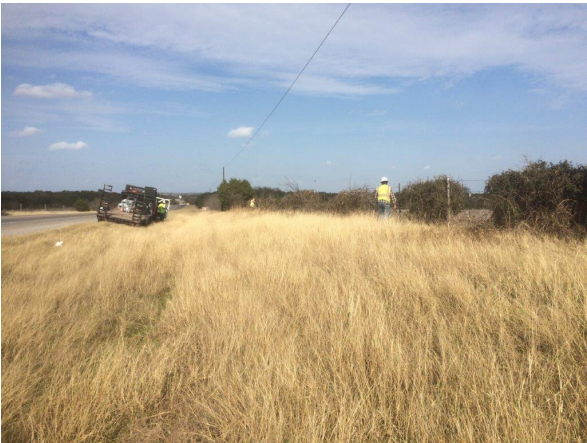
3. C-3 Environmental Fence Removal North of FM 2770 Eastside of FM 1626
