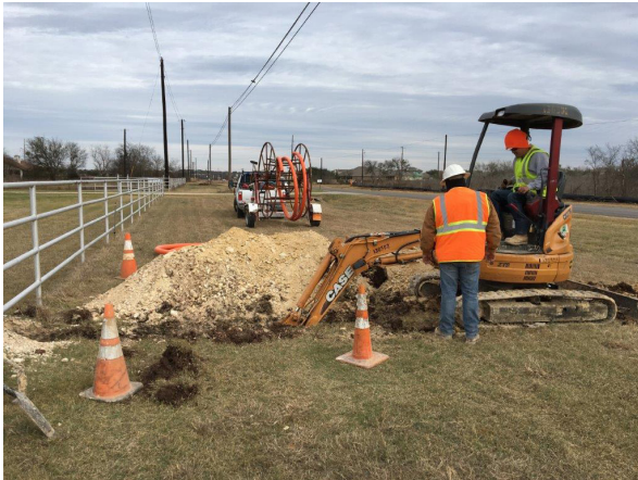
1. TWC Relocations South of Cold Water Hollow Westside of FM 1626
