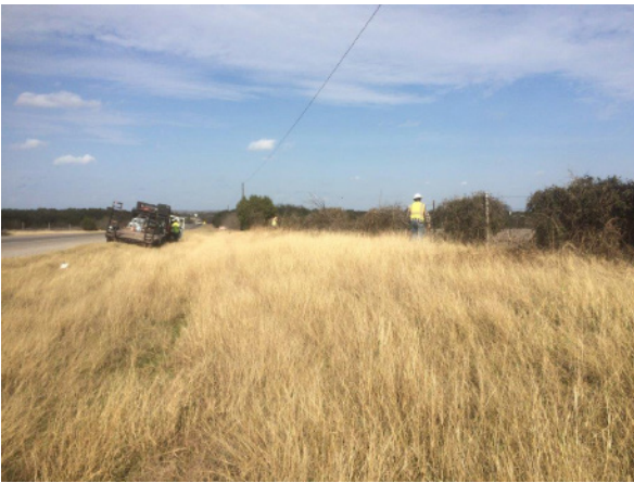
3. BMP Installing Silt Fence North of FM 2770
