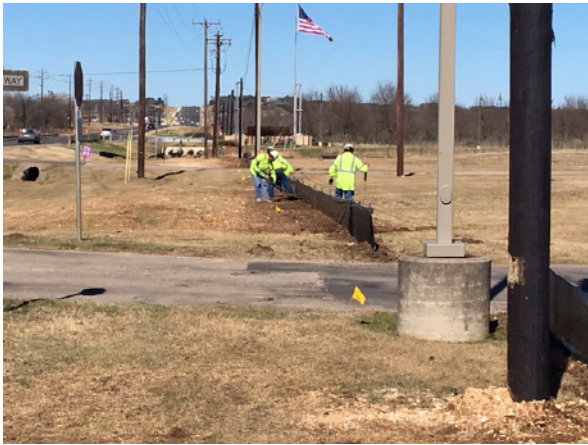
1. BMP Installing Silt Fence South of Oyster Creek
