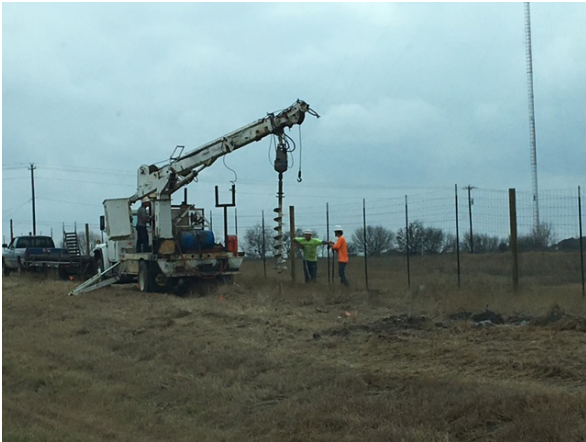
1. Frontier Installing Utility Poles North of FM 2770
