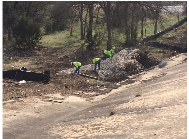
4. BMP Installing Rock Filter Dam N of Onion Crk (Culv 3 Downstream)
