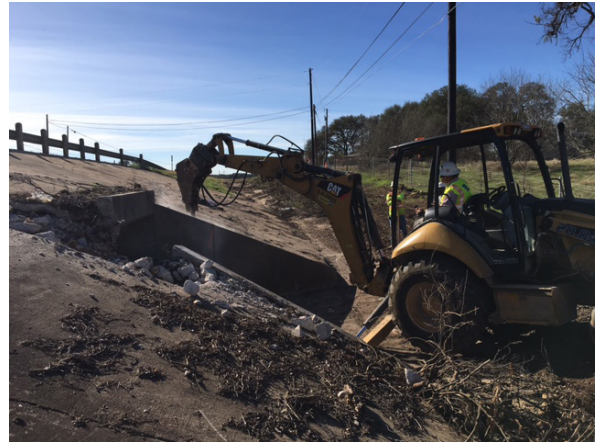
2. Sterling Removing Rip Rap N of Onion Crk (Culv 3 Upstream)
