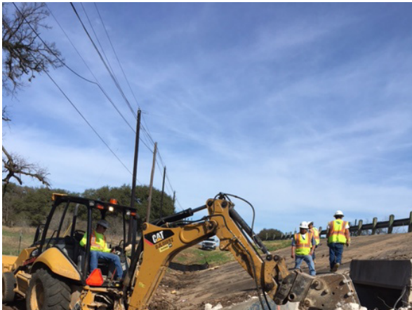
3. Sterling Removing Rip Rap N of Onion Crk (Culv 3 Upstream)
