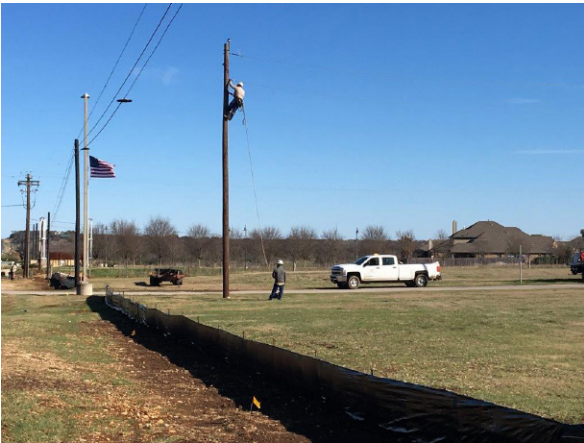
3. PEC Relocating and Removing Lines S of Oyster Creek
