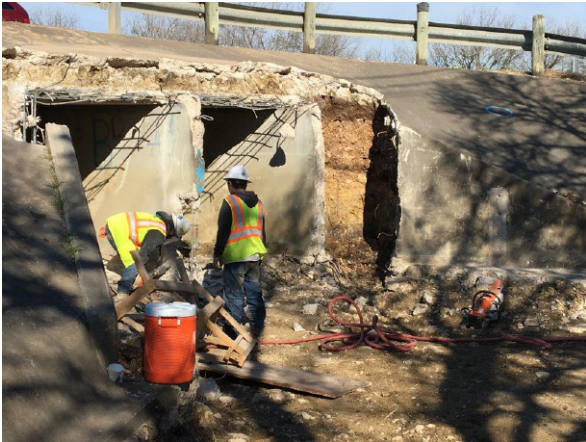
1. Sterling Removing Rip Rap S of Cole Springs Rd (Culv 4 Downstream)
