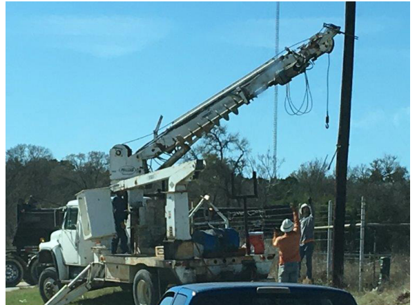
2. Frontier Installing Utility Poles N of FM 2770
