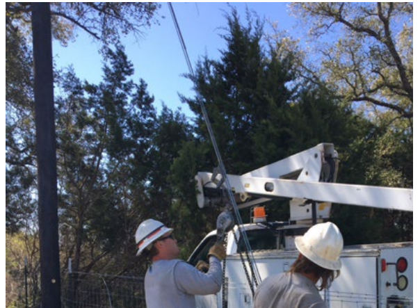
4. Frontier Installing Utility Pole N of FM 2770
