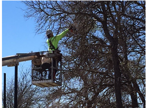
2. Frontier Trimming Branches for Span Wire N of FM 2770
