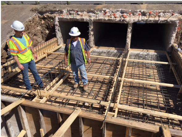
3. Sterling Forming & Placing Rebar N of Oyster Creek (Culvert 5 Upstream)
