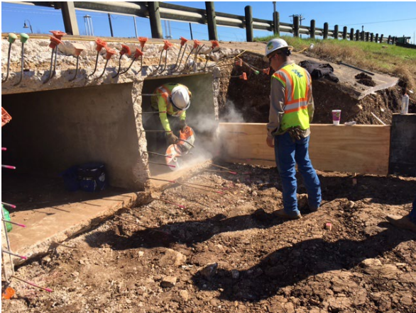
1. Sterling Sawcutting Existing Box Culvert N of Oyster Creek
