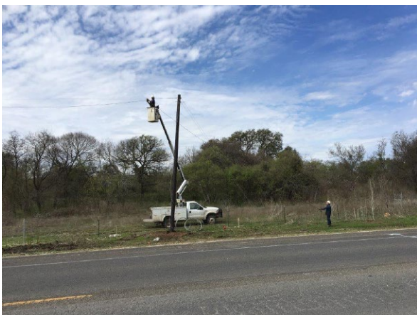
5. Frontier Installing Span Wire N of Onion Creek
