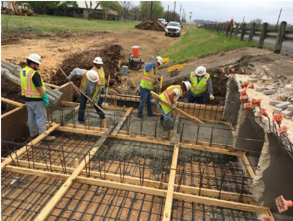
1. Sterling Pouring Footing on Existing Box Culv N of Oyster Creek
