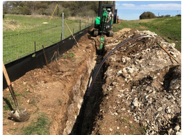
4. Zayo Group Installing Fiber Line N of Onion Creek
