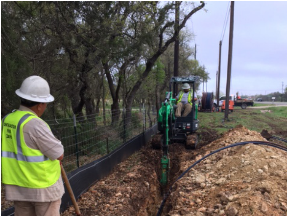
1. Zayo Group Installing Fiber Line S of Cold Springs Rd
