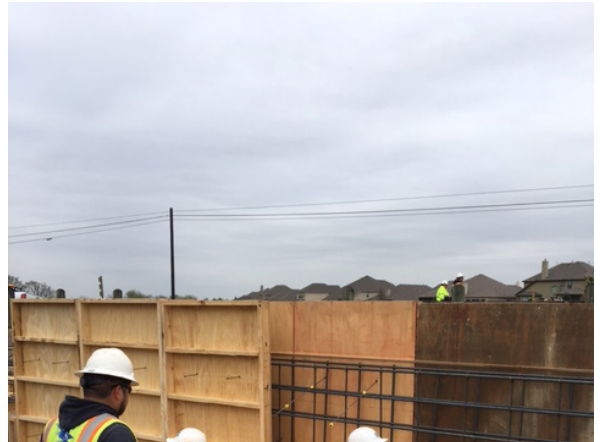
2. Sterling Forming Wall of Proposed Box Culv N of Oyster Creek
