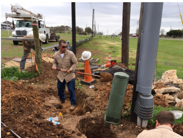
5. PEC Locating Existing Utility S of Oyster Creek
