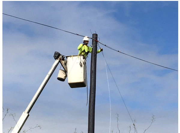
4. Frontier Installing Span Wire N of Onion Creek
