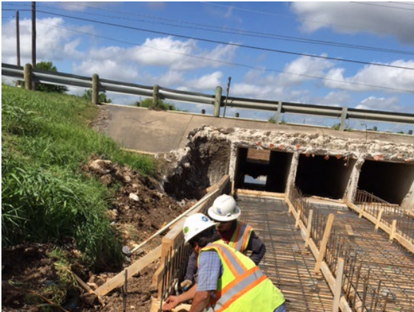
1. Sterling Placing Steel for Proposed Box Culv N of Oyster Crk
