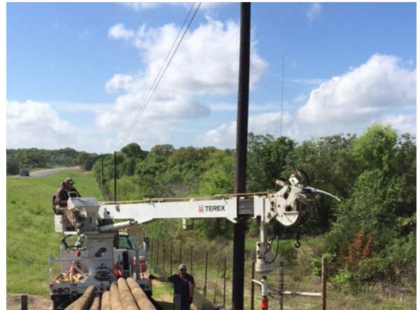
4. Zayo Installing Utility Pole N of Mustang Crk
