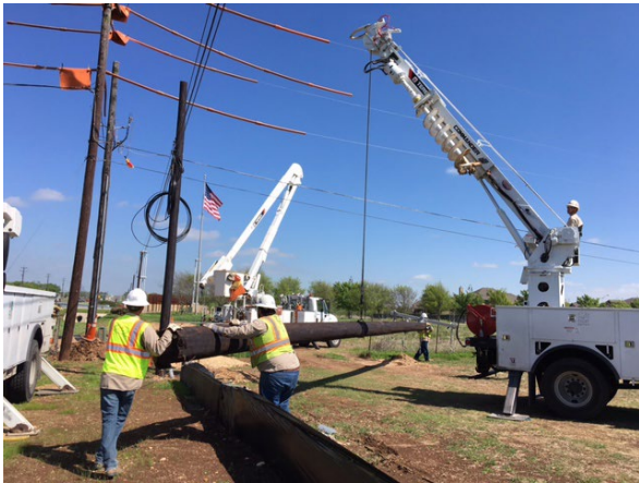
3. PEC Installing Utility Pole at Elm Grove Elementary
