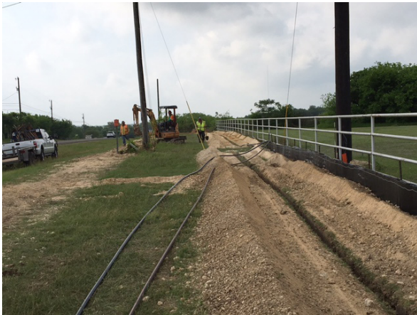
3. Zayo Installing Underground Utility at Old Black Colony
