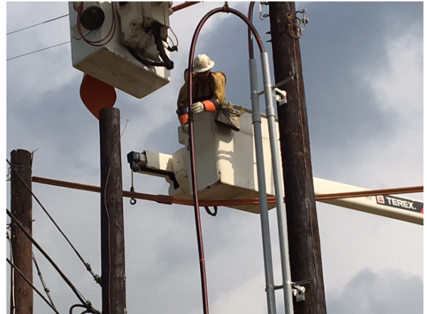
2. PEC Installing Proposed Utility at Elm Grove Elementary
