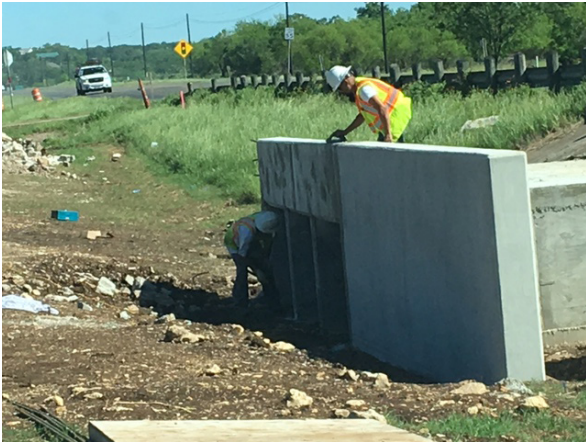
1. Sterling Patching Proposed Box Culver N of Oyster Crk
