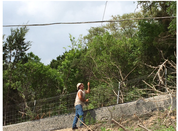
4. Zayo Installing Span Wire S of Mustang Crk
