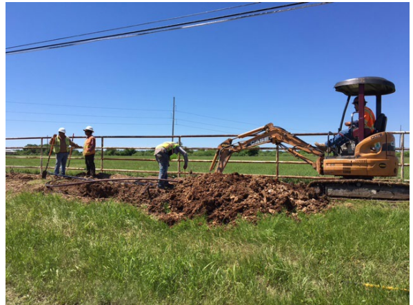
4. Zayo Installing Underground Utilities S of Hy Rd
