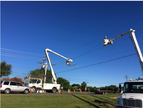
3. PEC Installing Span Wire at Oyster Creek Dr
