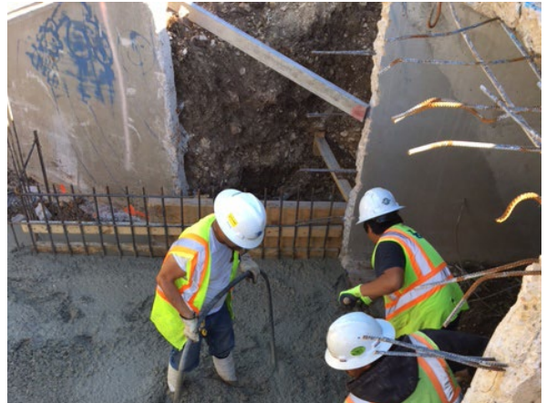
2. Sterling Pouring Concrete for Proposed Box Culv N of Onion Creek
