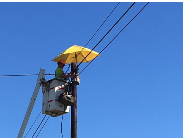
5. Frontier Splicing Connection N of Oyster Creek Dr
