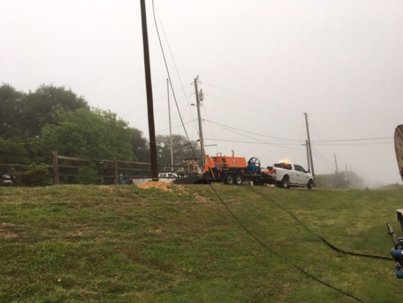
1. Zayo installing Span Wire N of Onion Creek
