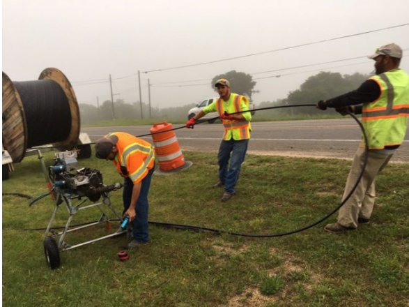
2. Zayo installing Span Wire N of Onion Creek
