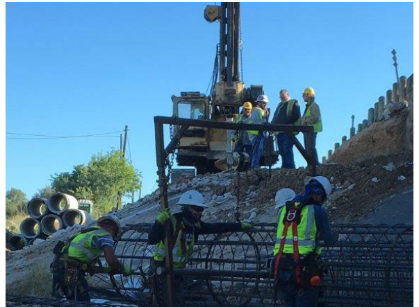
4. Sterling Tying Bridge Steel at Mustang Crk
