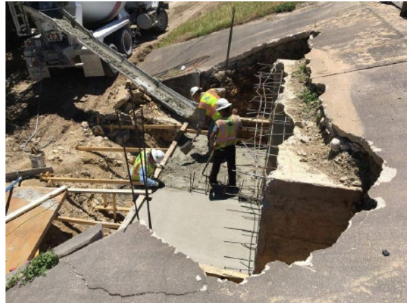
2. Pouring Bottom Slab of Box Culv S of Cole Springs
