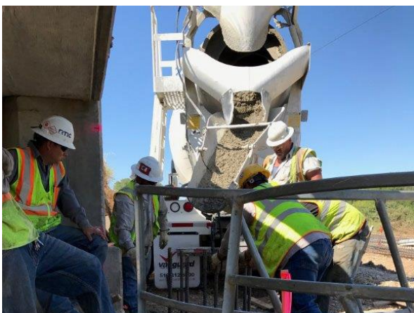
5. Sterling Pouring Drill Shaft on North End of Mustang Crk
