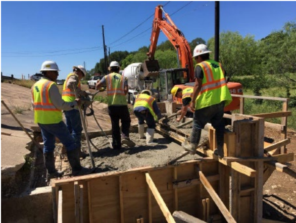
1. Pouring Top Slab of Box Culv N of Onion Creek
