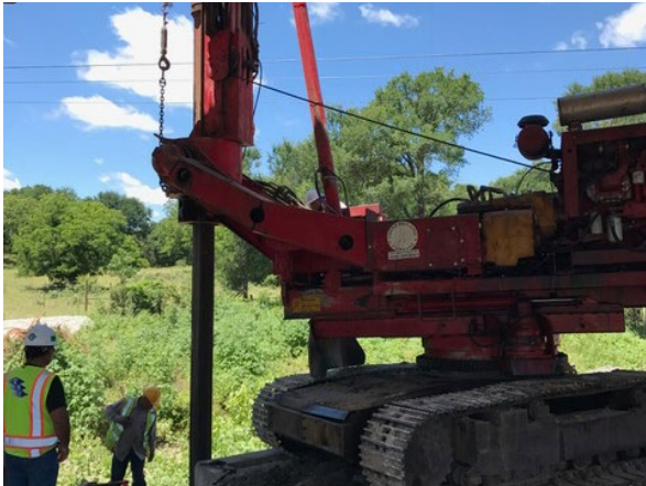
2. Sterling Drilling Shaft at Mustang Crk
