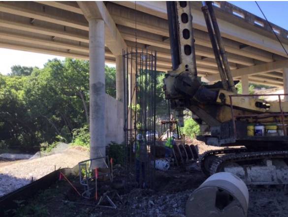
1. Sterling Lowering Drilled Shaft Cage at Mustang Crk
