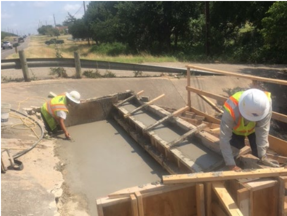
1. Finishing Concrete for DS Culv Extension N of Onion Crk
