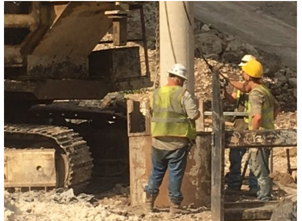
2. Drilling Shaft at Mustang Crk Bridge
