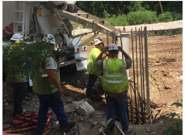
4. Pouring Drill Shaft at Mustang Crk Bridge
