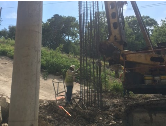
3. Placing Steel for Drill Shaft at Mustang Crk Bridge
