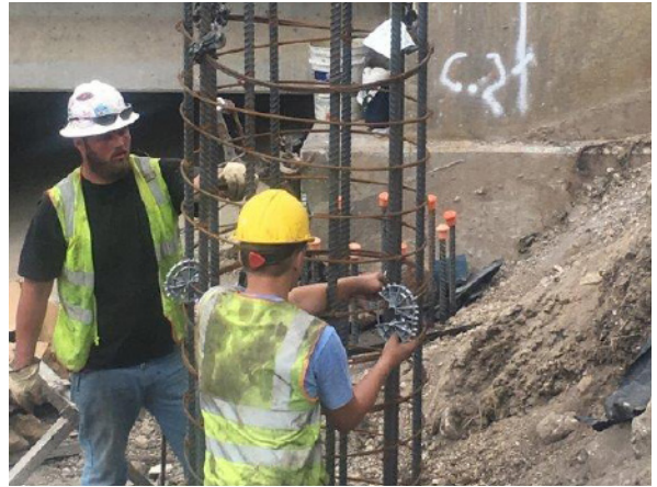
2. Sterling Lowering Drilled Shaft Cage at Mustang Crk
