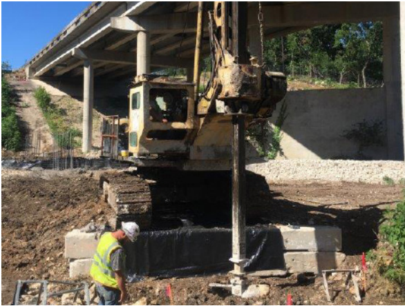
1. Sterling Drilling Shaft at Mustang Crk
