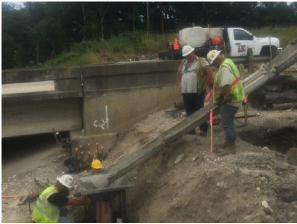
3. Sterling Pouring Drilled Shaft Concrete at Mustang Crk
