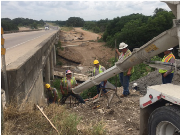
2. Sterling Pouring Drilled Shaft Concrete at Mustang Crk
