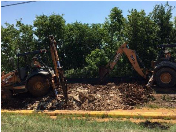
2. CenterPoint Trenching Gasline South of Old Black Colony
