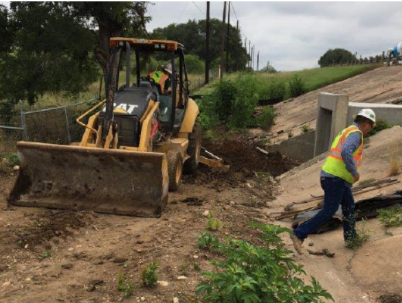
1. Sterling Performing Ditch Grading South of Cole Springs
