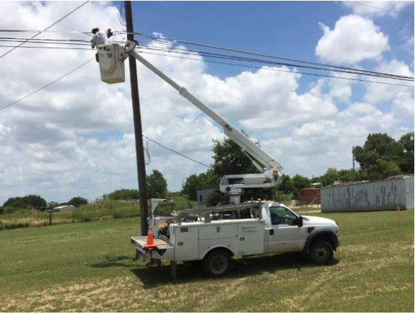
3. Spectrum Splicing Utility Lines N of Cole Springs
