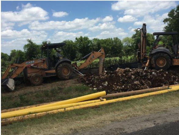
2. CenterPoint Gas Line Relocation S of Old Black Colony1
