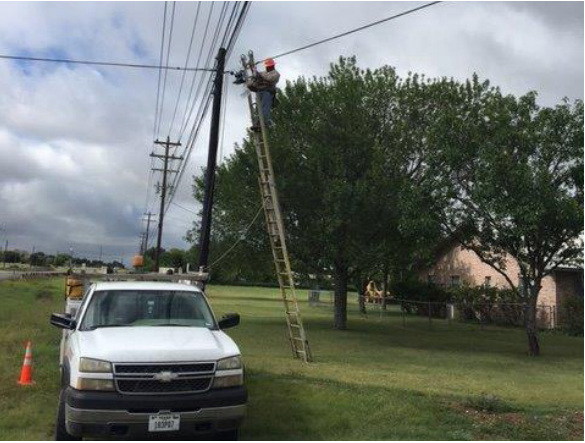
3. Frontier Splicing Utility W ROW Near Hy Rd
