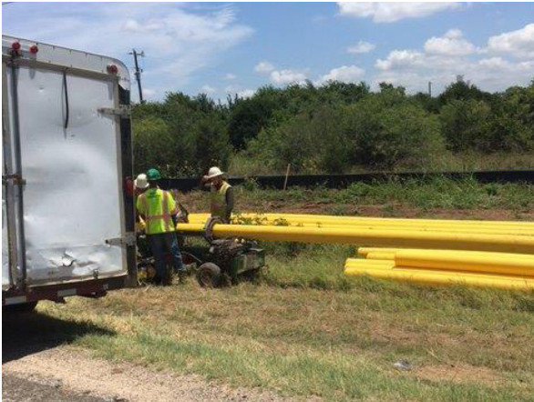
1. CenterPoint Fusing Pipe N of Onion Crk
