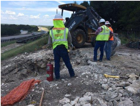
3. CenterPoint Relocating Gas Line S of Mustang Crk
