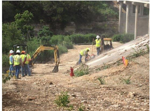
2. CenterPoint Removing Rip Rap at Onion Crk
