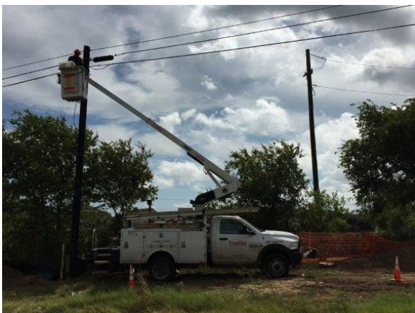
5. Frontier Splicing New Utility Line N of Old Black Colony
