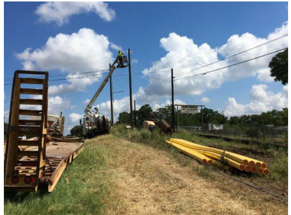
4. Spectrum Removing Old Utility Line N of Onion Crk
