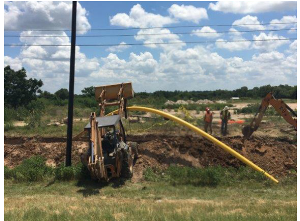
2. CenterPoint Installing Gas Line N of Onion Crk
