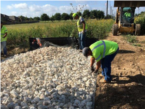
1. BMP Installing Rock Filter Dam N of Hy Rd
