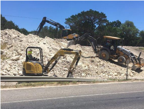
1. CenterPoint Installing Gas Line S of Mustang Crk
