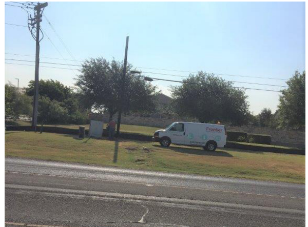
4. Frontier Splicing New Utility Line at Coldwater Hollow
