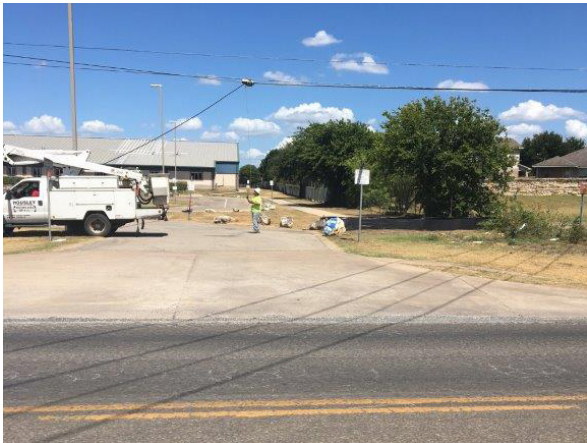
3. Spectrum Splicing New Utility Line N of Onion Crk
