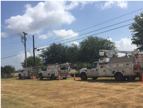
3. Frontier Installing New Span Wire S of Oyster Crk
