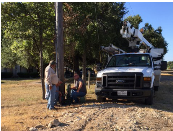
5. Frontier Splicing New Utility Line S of Old Black Colony Rd
