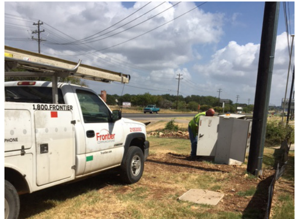
4. Frontier Splicing New Utility Line S of Oyster Crk
