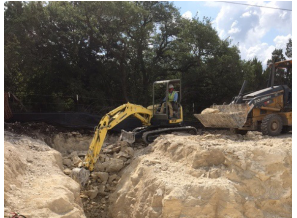
2. CenterPoint Installing Gas Line S of Mustang Crk
