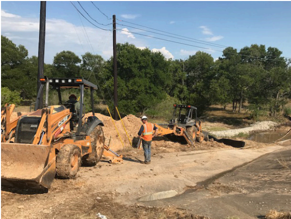
1. CenterPoint Installing Gas Line N of Onion Crk
