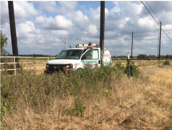
3. Frontier Splicing New Utility Line N of FM 2770
