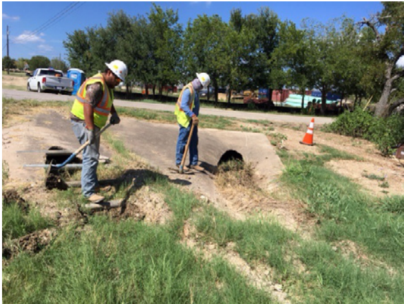
2. Sterling Maintaining Erosion Controls S of Cole Springs Rd
