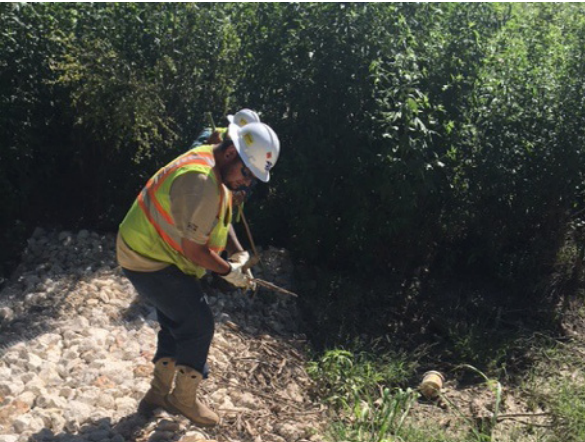
1. Sterling Maintaining Erosion Controls at Onion Crk
