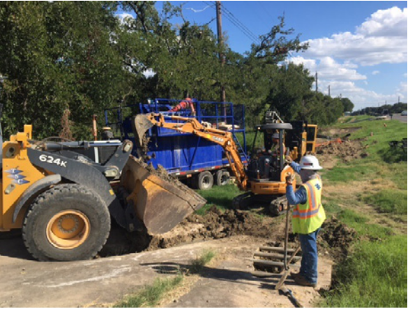
3. Sterling Maintaining Erosion Controls S of Cole Springs Rd
