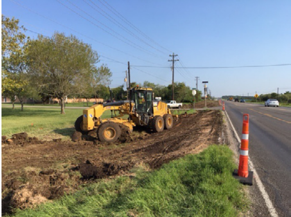
2. Sterling Striping Topsoil S of RM 967
