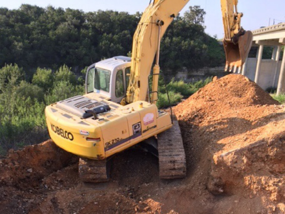
1. CenterPoint Installing Gas Line at Onion Creek
