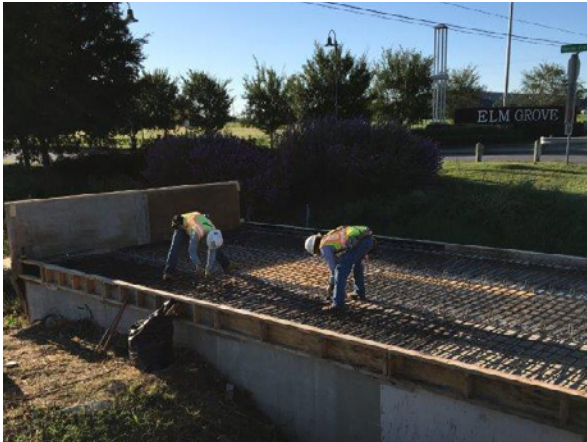
2. Sterling Tying Steel at Culvert 5 N of Oyster Crk
