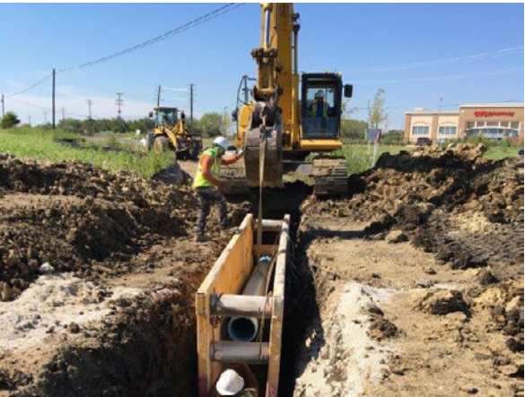
3. DC Civil Installing Waterline at RM 967
