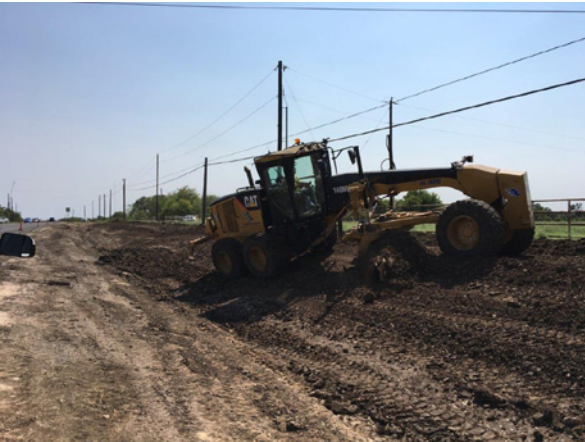
1. Sterling Stripping Topsoil N of Coldwater Hollow
