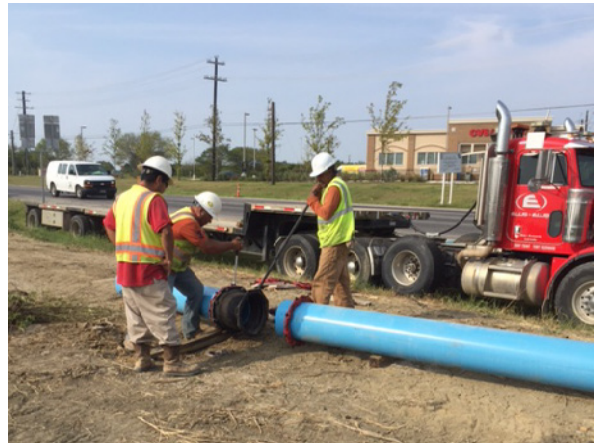
4. DC Civil Connecting Pipe for Waterline S of RM 967
