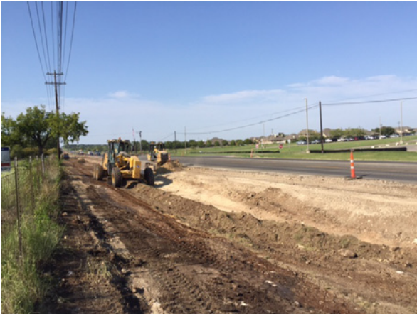
1. Sterling Embanking for Detours N of Coldwater Hollow
