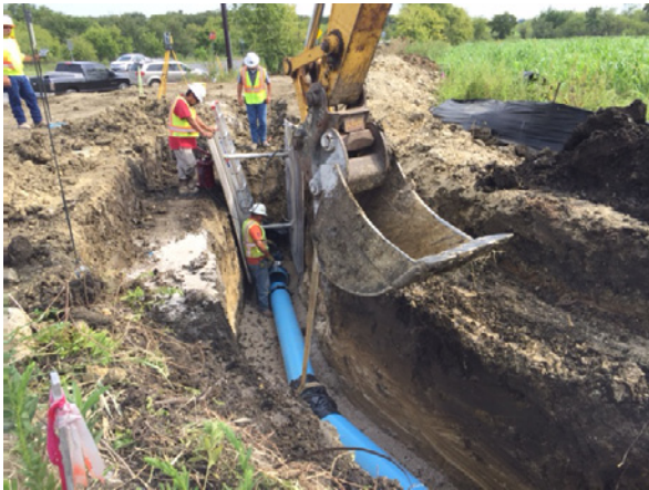
3. DC Civil Installing Waterline at RM 967
