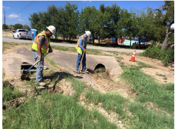
2. Sterling Demolishing Culvert 4 S of Cole Springs
