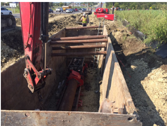
5. Ellis & Ellis Boring Waterline S of RM 967
