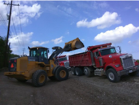
1. Sterling Hauling Topsoil N of Hy Rd
