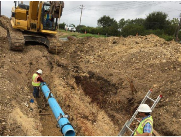
3. DC Civil Installing Waterline S of Oyster Creek
