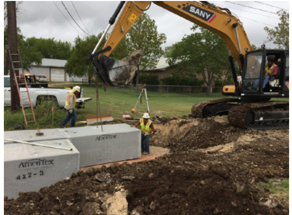
2. Sterling Placing Driveway Drainage Culvert N of Oyster Crk Dr
