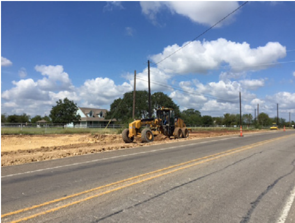
1. Sterling Grading Detour N of Cole Springs
