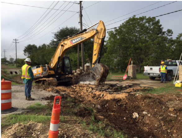
3. Sterling Removing Existing Driveway Drainage Culvert N of Oyster Cree...
