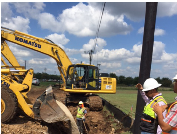
5. DC Civil Installing Waterline S of Oyster Creek
