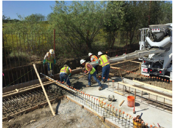
2. Sterling Pouring Wingwall Slab for Upstream Culv 4
