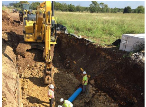
4. DC Civil Installing Waterline S of Oyster Creek
