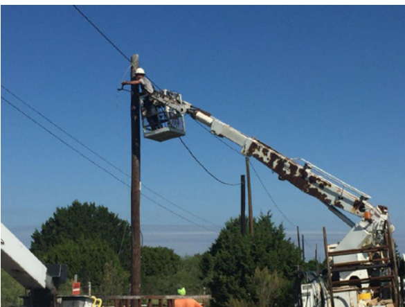
5. Frontier Wrecking Utility Lines by N. of Mustang Creek
