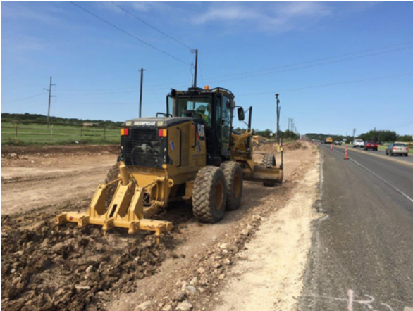
1. Sterling Grading Detour N of Cole Springs
