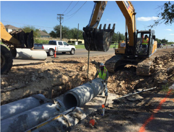
3. Sterling Installing Driveway Culvert N of Oyster Creek
