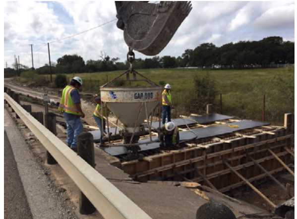
2. Sterling Pouring Walls on Culv 4 Upstream
