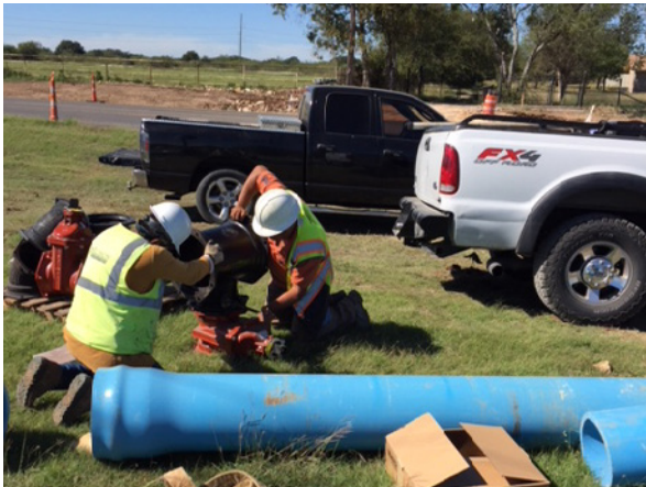
3. DC Civil Prepping Waterline for Installation
