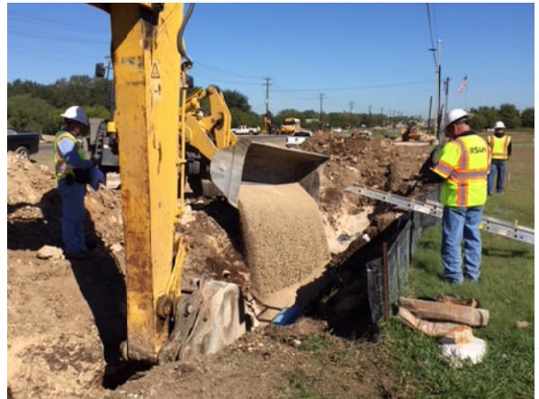
4. DC Civil Backfilling Waterline S of Oyster Creek
