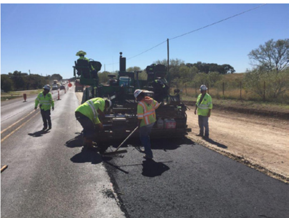
5. Austin Material Paving Temp. Widening N of Cole Springs
