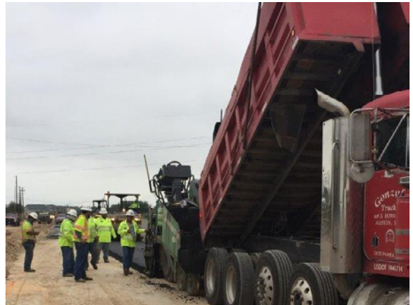
4. Austin Material Paving Temp. Widening S of Oyster Creek
