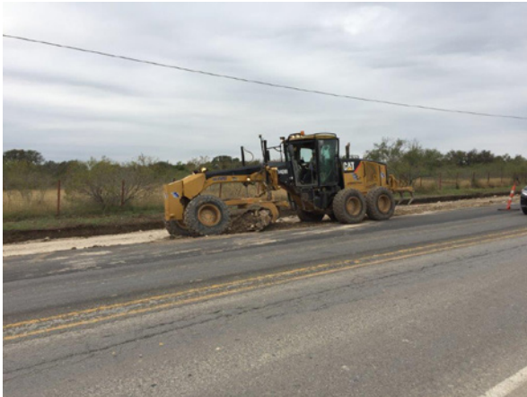
1. TSC Placing Shoulder on Temp Widening N of Cole Springs
