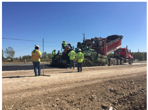
6. Austin Material Paving Temp. Widening N of Cole Springs
