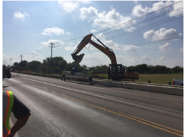
2. TSC Installing LPCB at Oyster Crk
