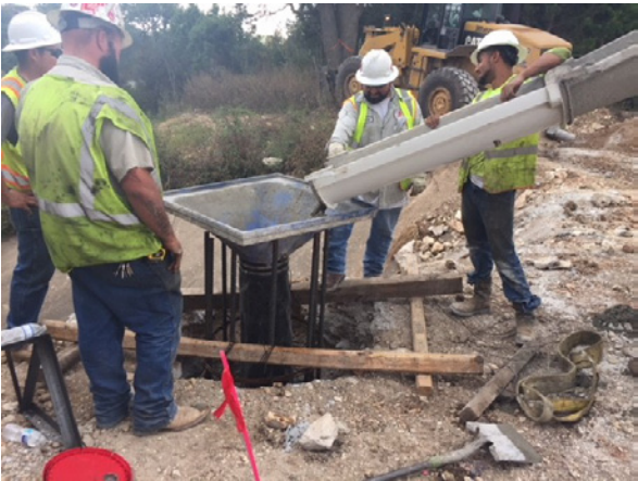
3. Voges Pouring Drilled Shaft at Abut 7 Onion Crk
