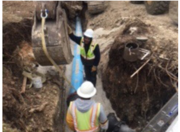
2. DC Civil Installing Waterling at Oyster Crk Dr
