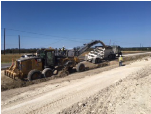
1. Sterling Milling Existing Roadway N of FM 2770
