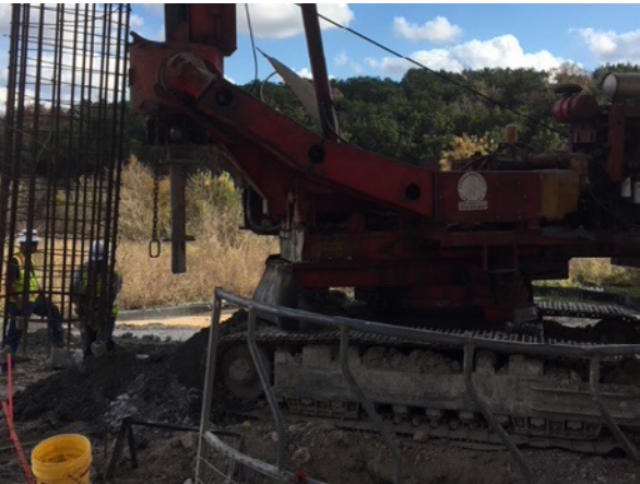
3. Voges Placing Steel for Bent 5 Drilled Shaft at Onion Crk
