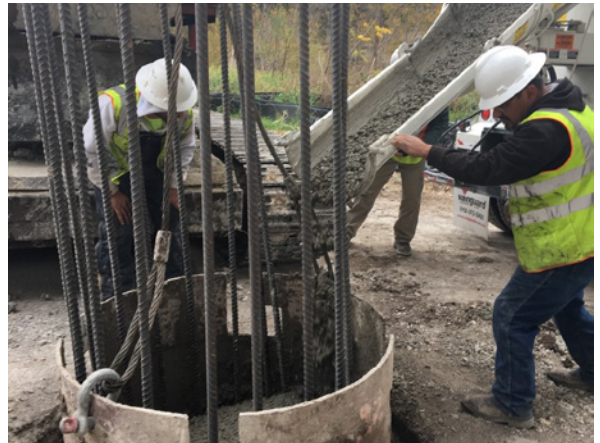
4. Voges Pouring Drilled Shaft for Bent 5 at Onion Creek
