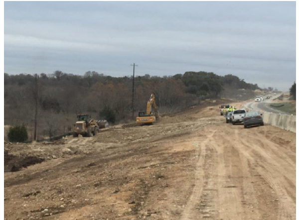
2. Sterling Performing Earthwork Operations N of Mustang Crk
