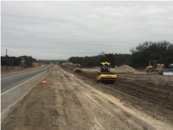
1. Sterling Performing Earthwork Operations N of FM 2770
