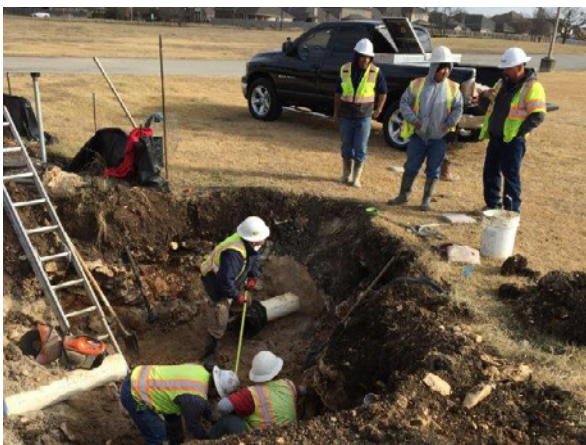
5. DC Civil Installing Tie-in for WL-A at Elm Grove Elementary
