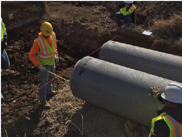
3. Sterling Installing Stormwater Drainage N of Oyster Crk Dr
