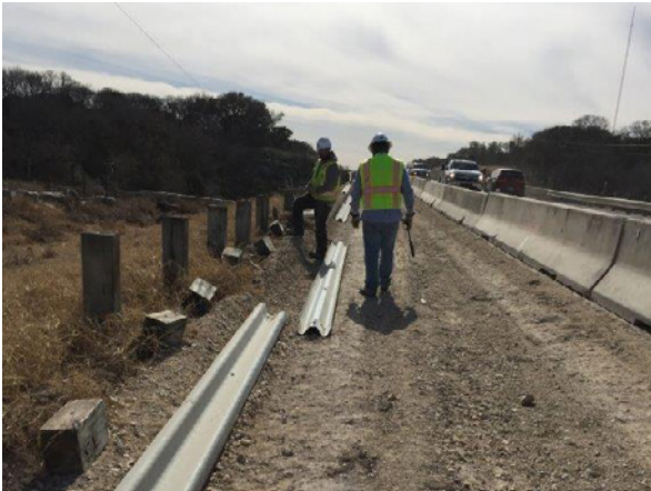
1. Sterling Removing MBGF N of Mustang Crk Bridge
