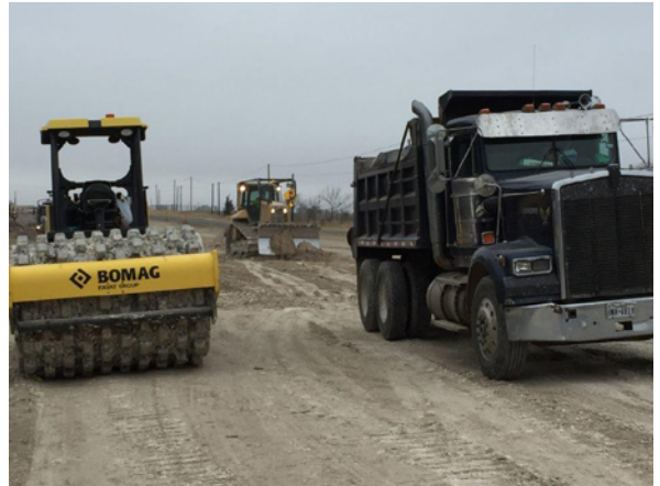
2. Sterling Performing Earthwork Operations N of FM 2770
