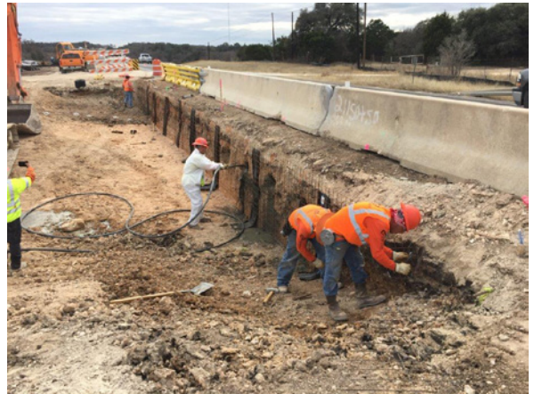
4. Subcontractor Orduno Constructing Temp Shoring Walls
