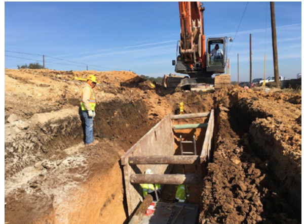
4. Sterling Placing 4x2 Culvert N of Onion Crk
