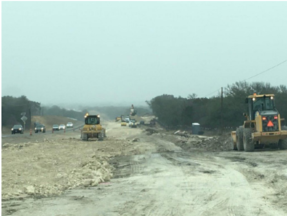
1. Sterling Performing Earthwork Operations S of Mustang Crk
