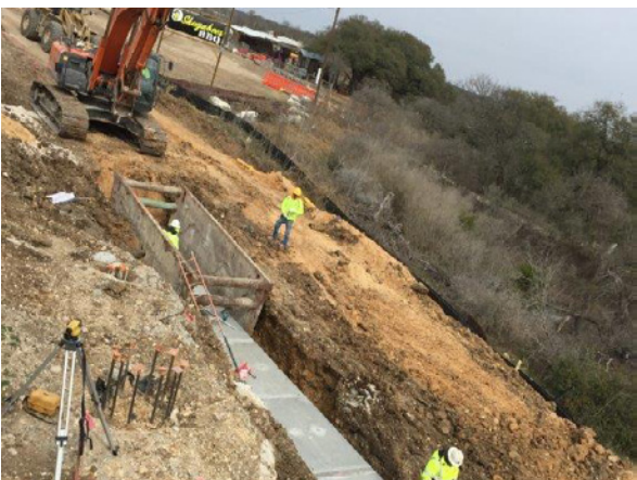
5. Sterling Placing 4x2 Culvert N of Onion Crk
