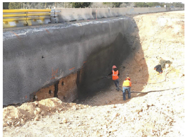
6. Oscar Orduno Placing Temp Shoring N of Mustang Crk
