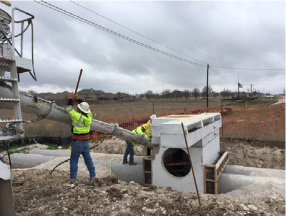
3. Sterling Pouring Collar at Culv 6 N of Oyster Crk
