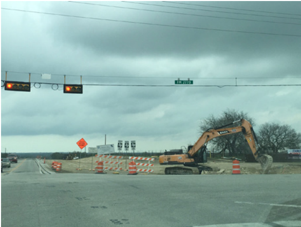
1. Sterling Performing Earthwork Operations at FM 2770
