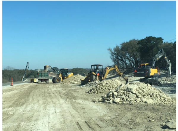
2. Sterling Performing Earthwork Operations S of Mustang Crk
