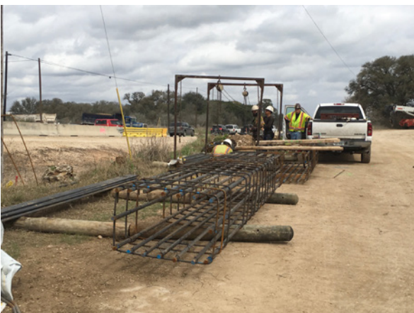
5. Breda Tying Steel for Abutment 7 at Mustang Crk
