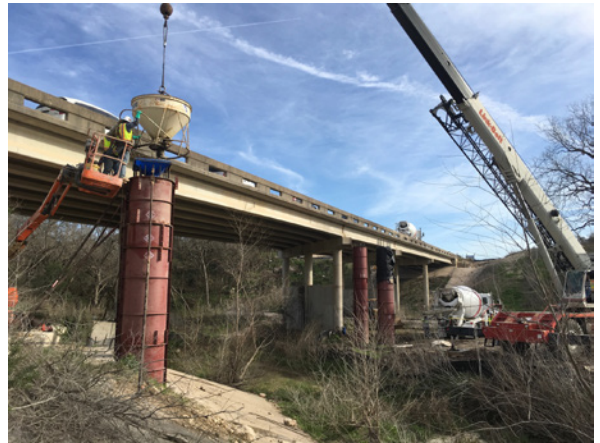
4. Sterling Pouring Columns at Mustang Crk
