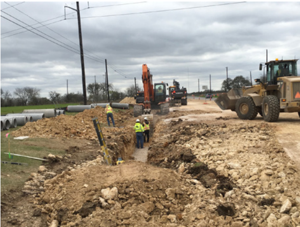
3. Sterling Installing Drainage System 2 N of Old Black Colony
