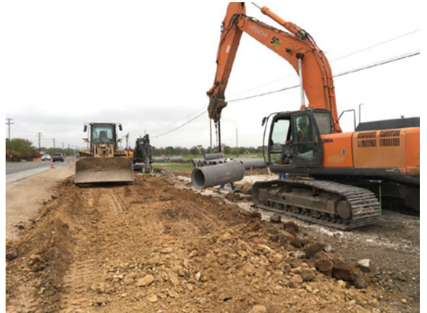
4. Sterling Placing Pipe N of Oyster Creek
