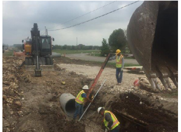
2. Sterling Placing Drainage Pipe N of Coldwater Hollow
