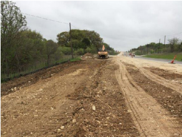
1. Sterling Earthwork Operations N of Mustang Crk
