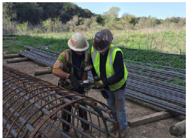
6. Breda Tying Steel at Onion Crk
