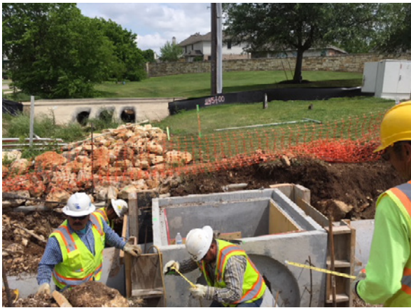
1. Sterling Placing Drainage Inlet N of Oyster Creek
