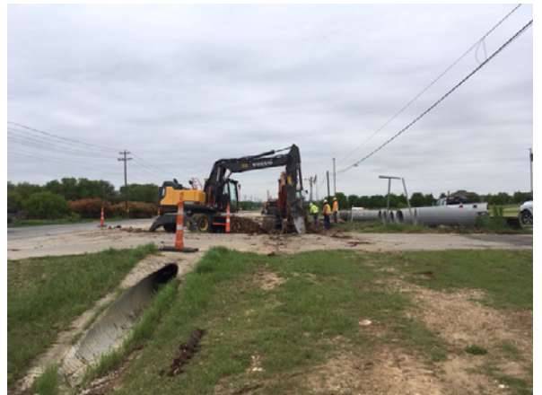
2. Sterling Placing Drainage Pipe N of Oyster Creek
