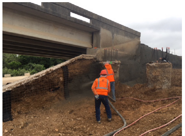
6. Oscar Orduno Constructing Temp Shoring at Mustang Crk
