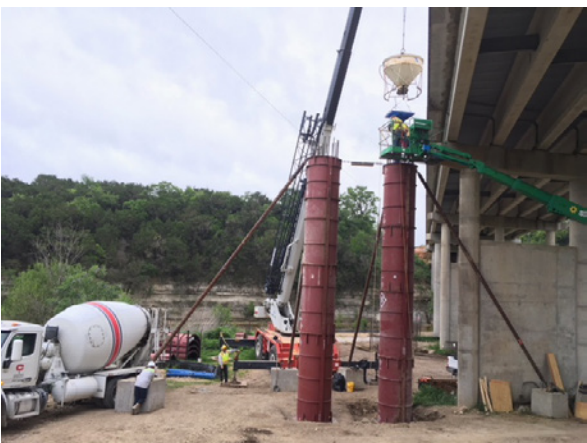
5. Sterling Pouring Columns at Onion Crk
