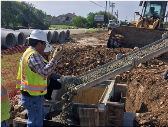
1. Sterling Pouring RCP Collar N of Oyster Creek
