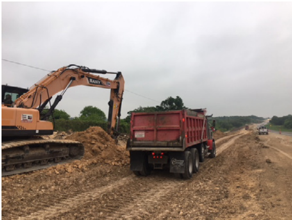
3. Sterling Earthwork Operations N of Mustang Crk
