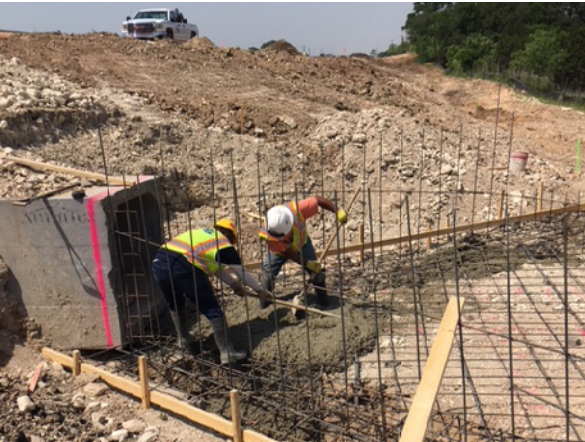
7. Sterling Pouring Slab for Culv 1
