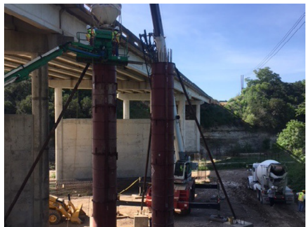
6. Sterling Pouring Columns at Onion Crk
