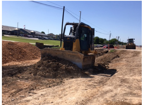
4. Sterling Earthwork Operations S of Oyster Creek
