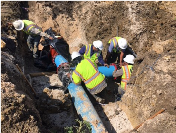
8. DC Civil Completing Tie-in N of Hy Rd
